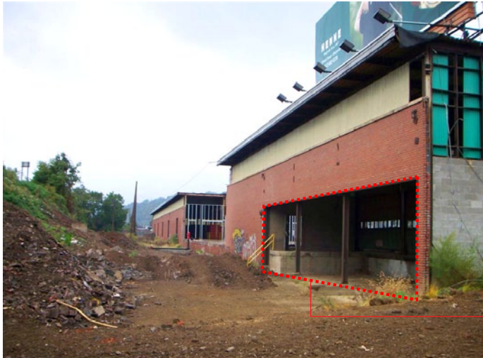
original south facade
