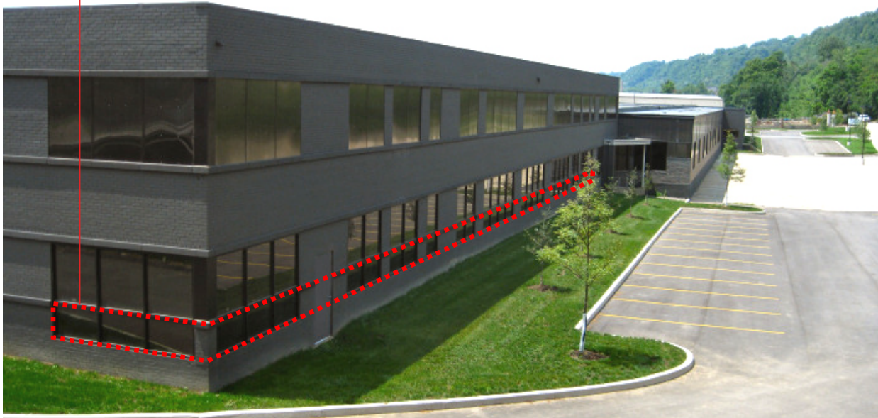
renovated north facade
