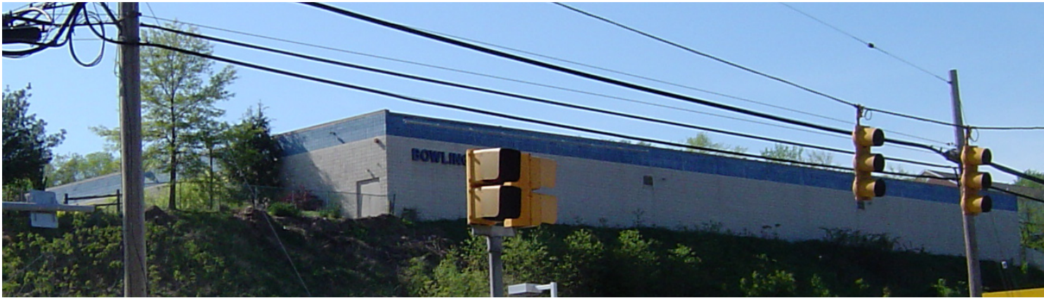
view from southeast prior to renovation
