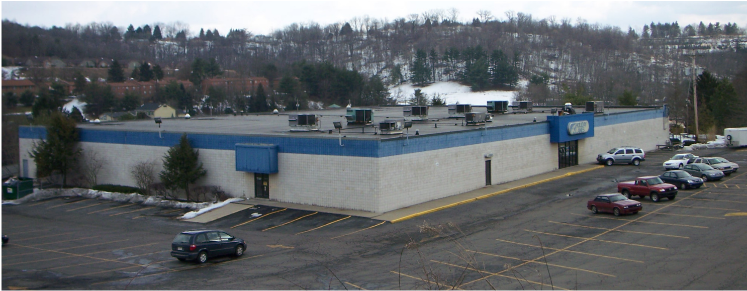
view from northwest prior to renovation
