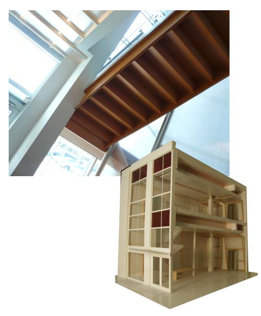
The new lobby serves all of the building tenants. A former exit stair was transformed into a main stair by enlarging the surrounding space and creating new guardrails and handrails. The creative use of finishes including a glowing polycarbonate ceiling and guardrail, sleek wood panelling, and terrazo flooring enhances the space.
